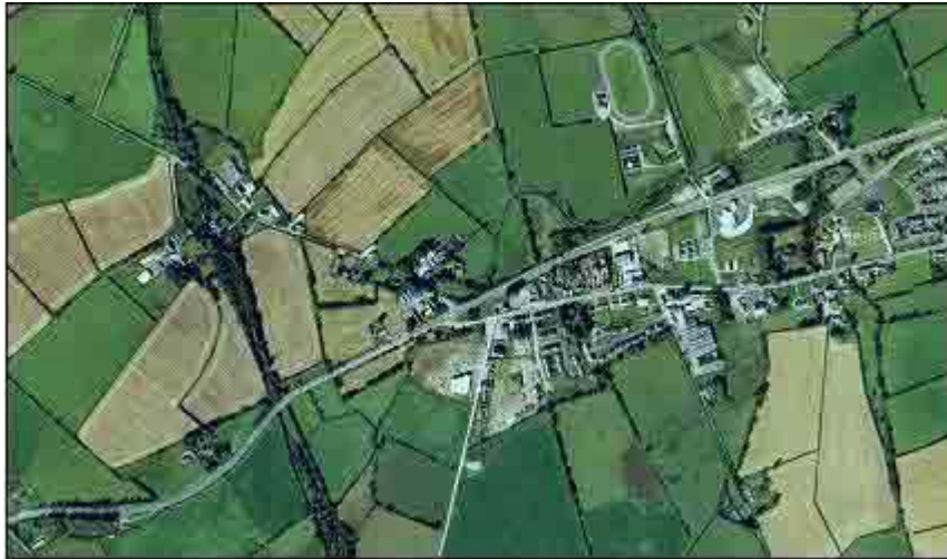
Figure 3. Aerial Photograph of Newtowncunningham 2004
